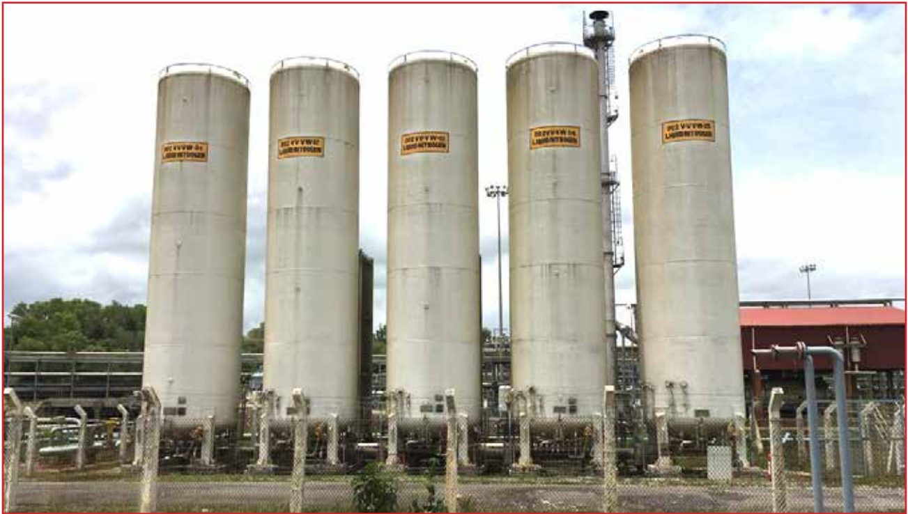
Nitrogen vessels used for maintaining inert atmosphere in Padur Caverns
