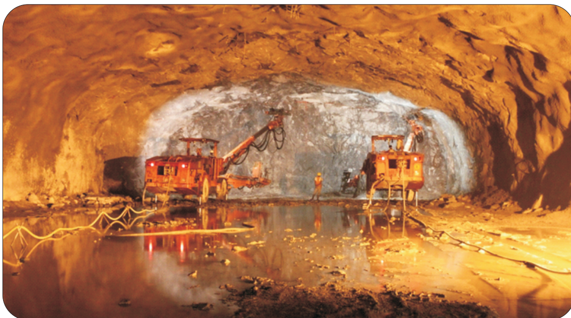
Cavern Top Heading under excavation at Mangalore
