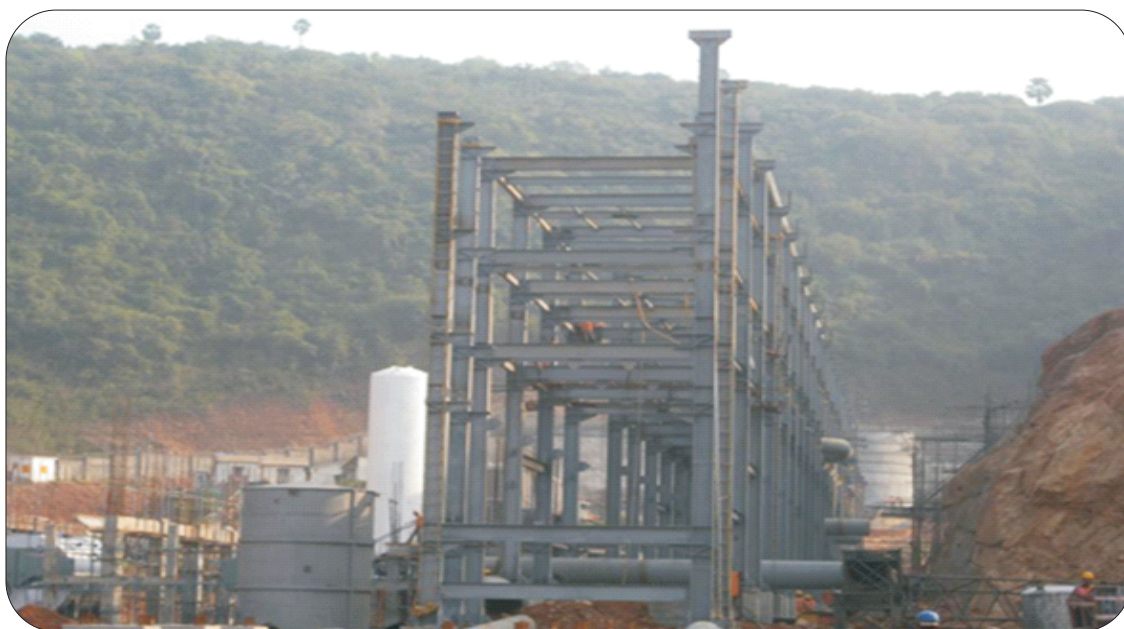
Pipe Rack under construction at Visakhapatnam site
